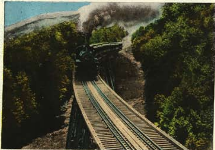
M. C. R. R. TRAIN CROSSING FRANKENSTEIN TRESTLE.
